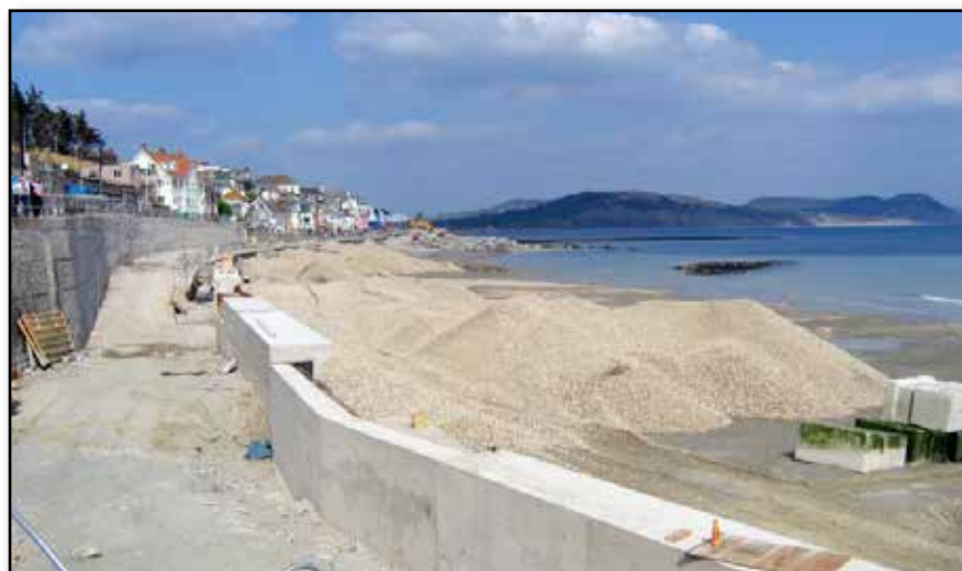
Figure 4: New sea wall and beach replenishment at Lyme
