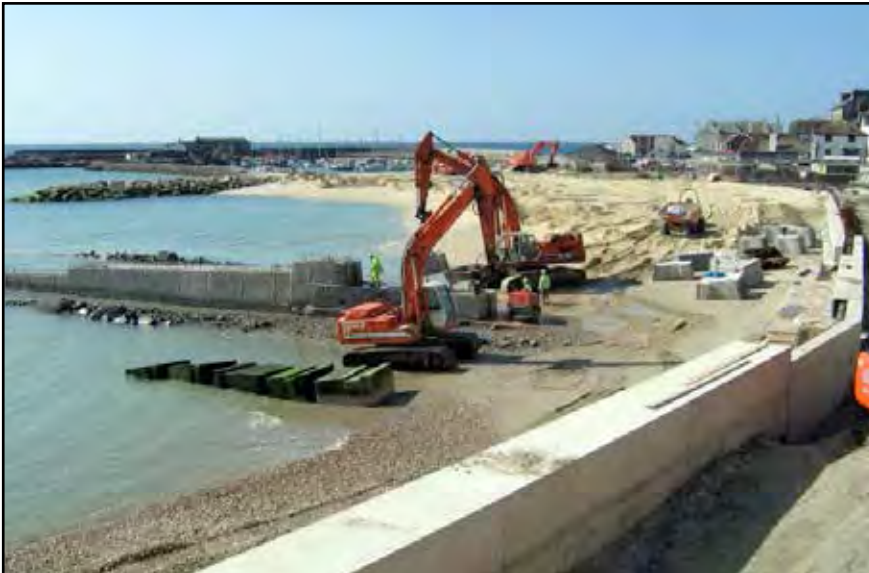
Figure 5: New sea wall, new groynes and replenishment beach at Lyme
